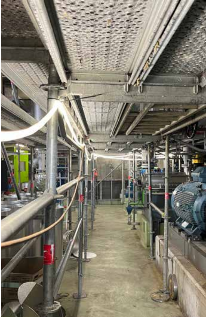
Scaffolding lighting, recycling plant
