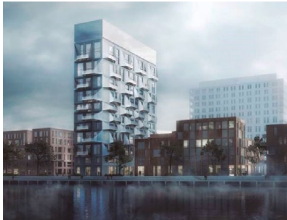
Denmark. The Silo
