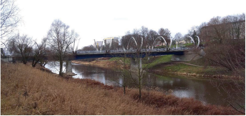
Figure 99: The Valmiera City Bridge over the Gaija River. Note the significant heights of the two embankments of the river and the steepness of the incline on both sides.
