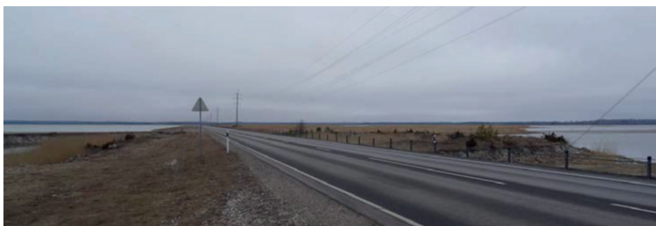
Figure 71: While maps tend to depict Saaremaa being connected by Muhu by a bridge, it is actually a causeway that has been constructed through marshland between the two islands. Therefore, this land transportation link would be far more difficult to cut than it would be to take down a bridge. Another implication is that it is impossible to travel via water directly from the Gulf of Rīga and the Väinameri.
