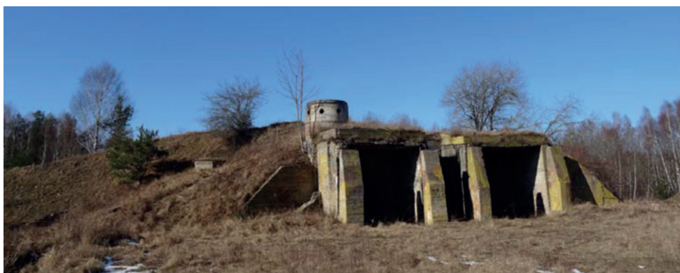
Figure 63: Surface-to-Air Missile (SAM) complex near the town of Piiri, on the island of Muhu. Note that the SAM TEL bunker was equipped with a pillbox, anticipating an attack by ground forces.
