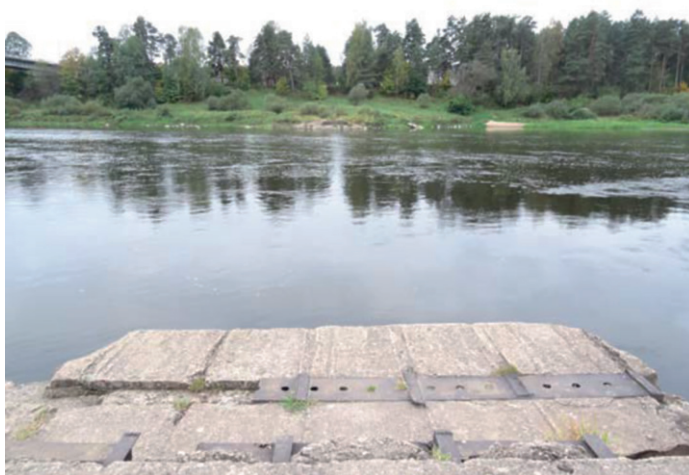
Figure 36: At a number of places, it was apparent that the Soviets had expected the interdiction of bridges and had, as a result, placed abutments for pontoon bridges (as was the case at Krāslava near the A6 bridge over the Daugava River) or concrete beds in the river to support movement in the event that bridges were made unusable in the course of conflict.
