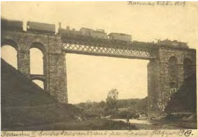
Estonian Armoured Train on Bridge over Raunas River between Lode Station and Cesis during the Landeswehr War. Source: Latvian War Museum Collection.
