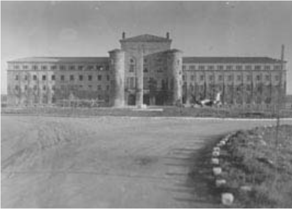
Fig. 9. Historical picture of the main building of the Ecole de l'air .
