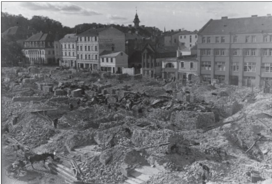
The damaged town centre south of the river.
