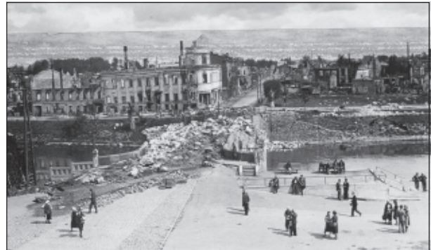
... from the same place after the demolition.
