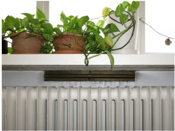
Slotted vent under a window. Photos: Netta Böök
