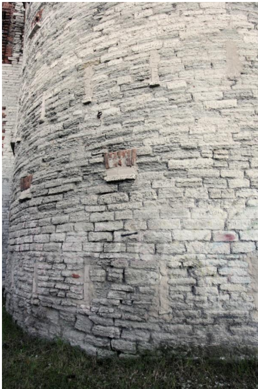
18. Half-tower in the eastern wing of the gorge, seaward façade. Bricked-up gun ports and smoke channels, curved bricked-up windows on sides of all three floors.
