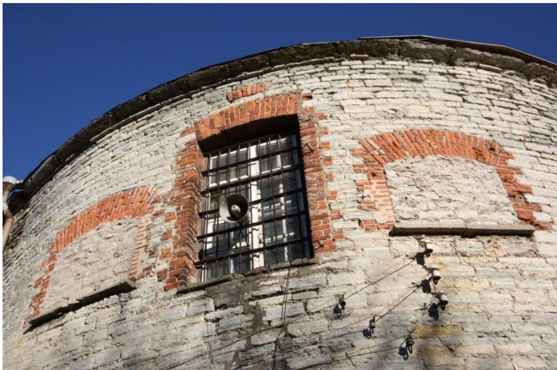
40. Curved end façade of the eastern wing of the gorge, on the 3 rd floor two preserved bricked-up embrasures and lintel of the smoke channel over a later window. Megaphone on the window.
