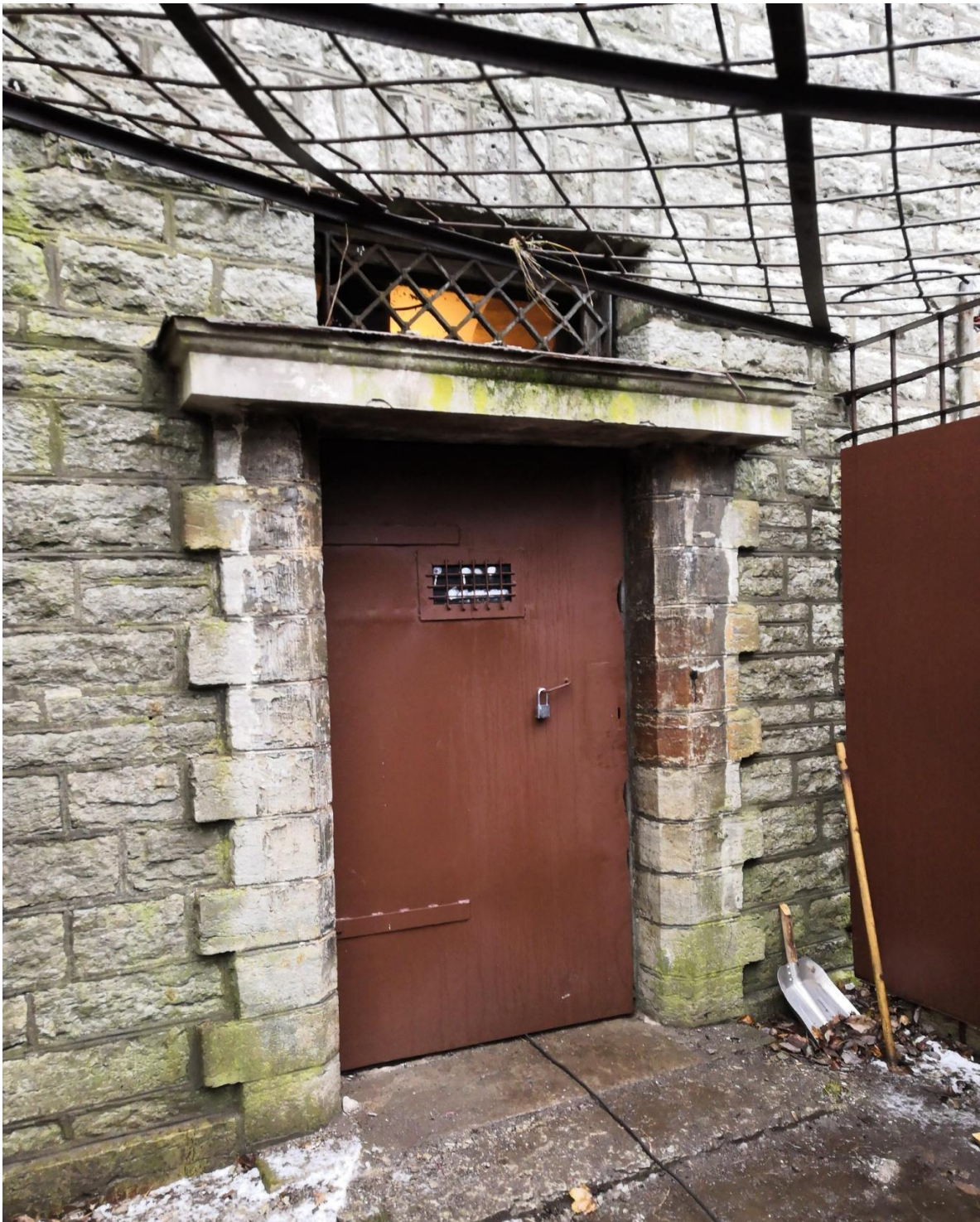
7. South-west façade door portal of the individual chamber building
