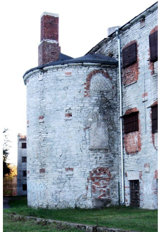
18. Half-tower in the eastern wing of the gorge, seaward façade. Bricked-up gun ports and smoke channels, curved bricked-up windows on sides of all three floors.
