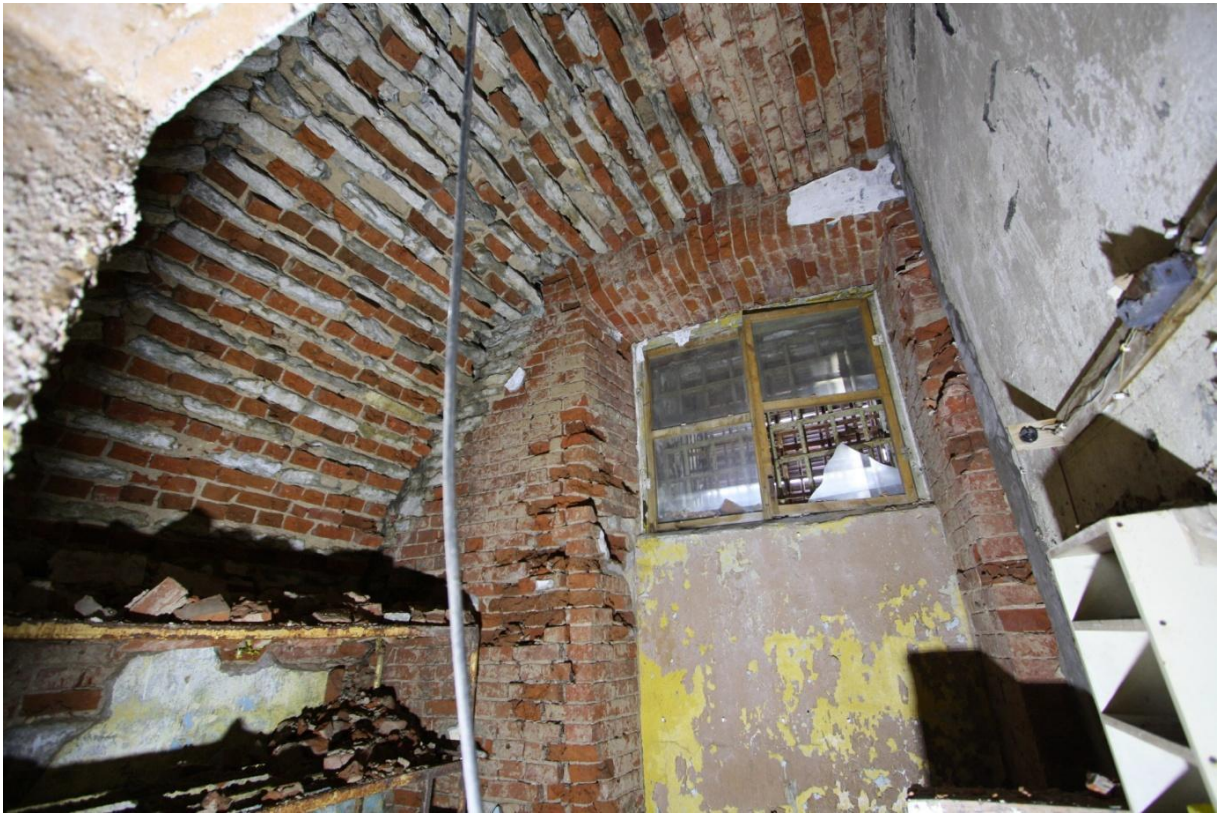
Photo 493. 3 rd floor auxiliary room
