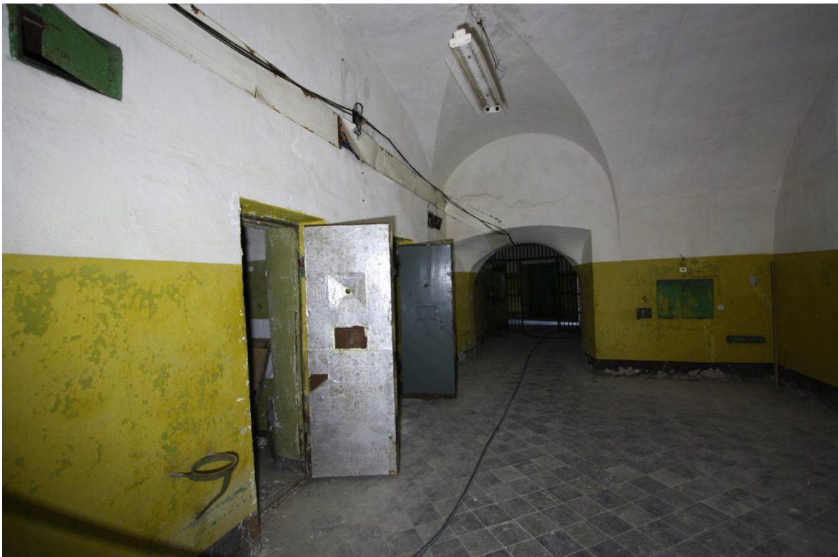
Photo 68. 2 nd floor corridor
