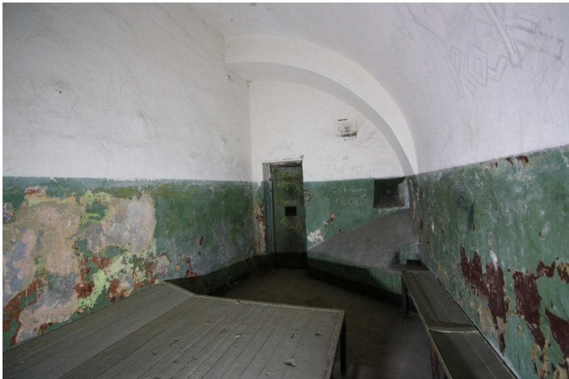
Photo 281. 2 nd floor cell
