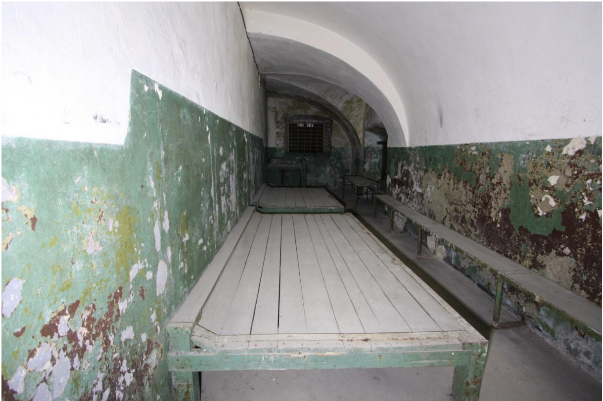
Photo 284. 2 nd floor cell
