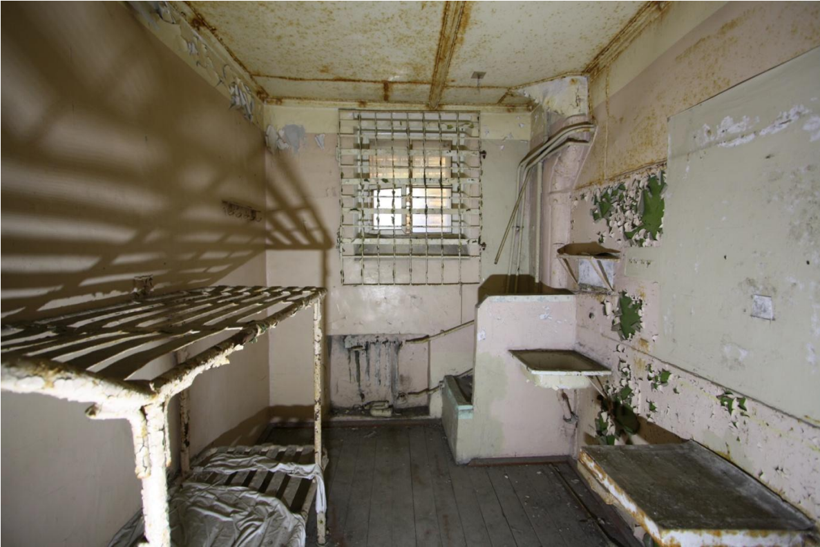
Photo 366. 3 rd floor cell
