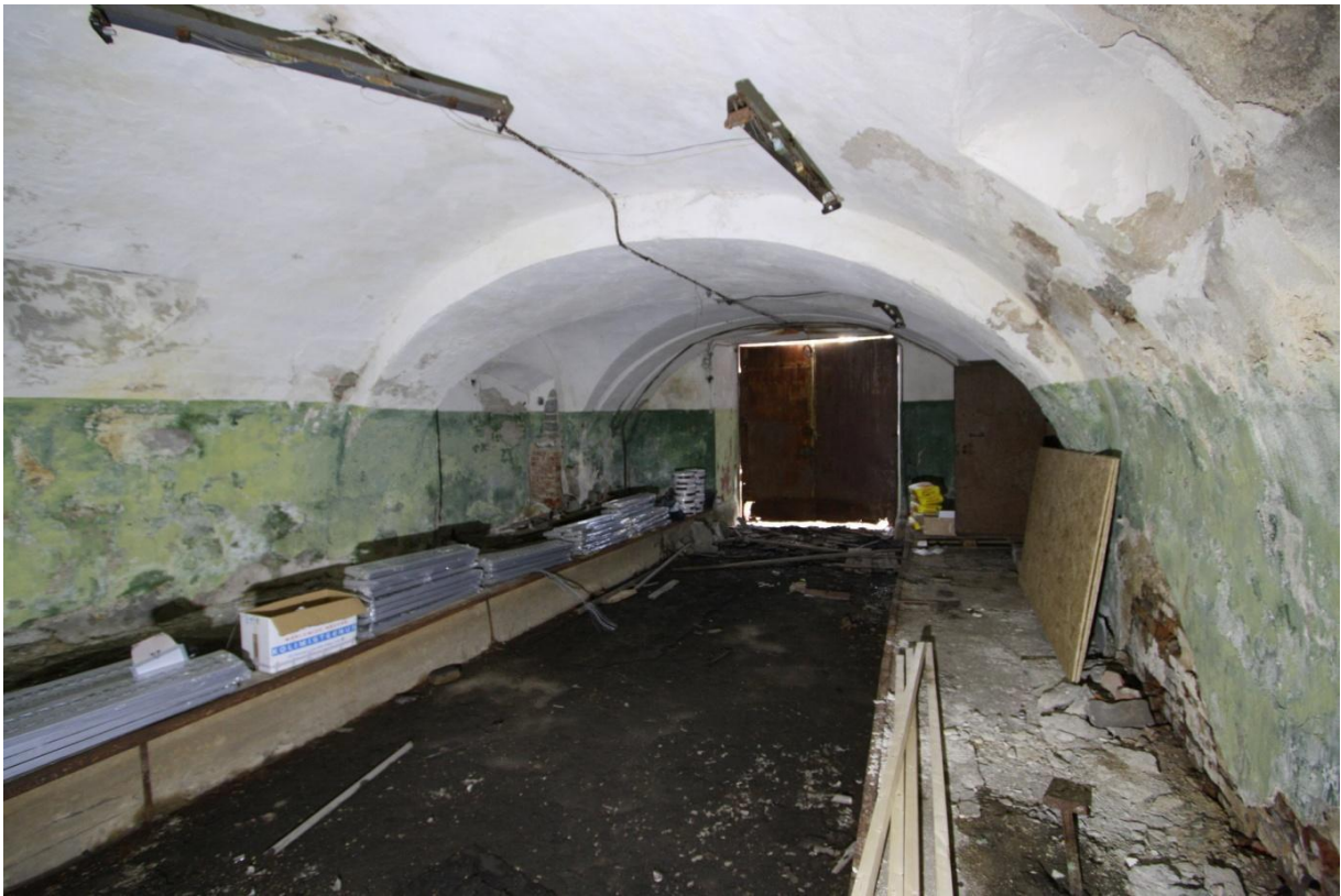
Photo 519. 1 st floor garage
