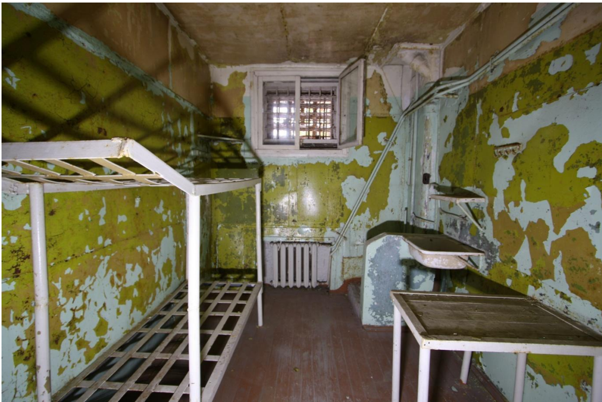
Photo 349. 2 nd floor cell
