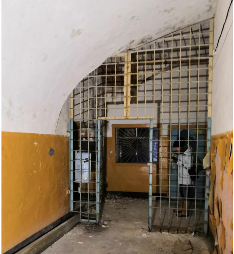
Photo 22. 2 nd floor corridor
