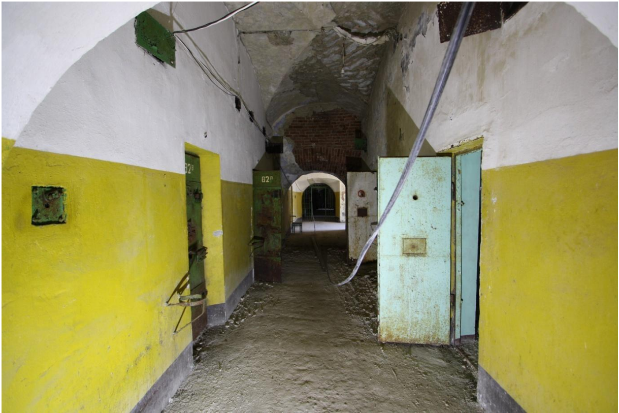
Photo 22. 2 nd floor corridor
