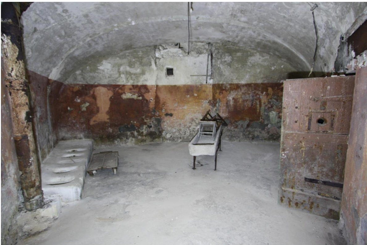
Gorge 2 nd floor sector 1 Photo 311. 2 nd floor prisoners' washroom
