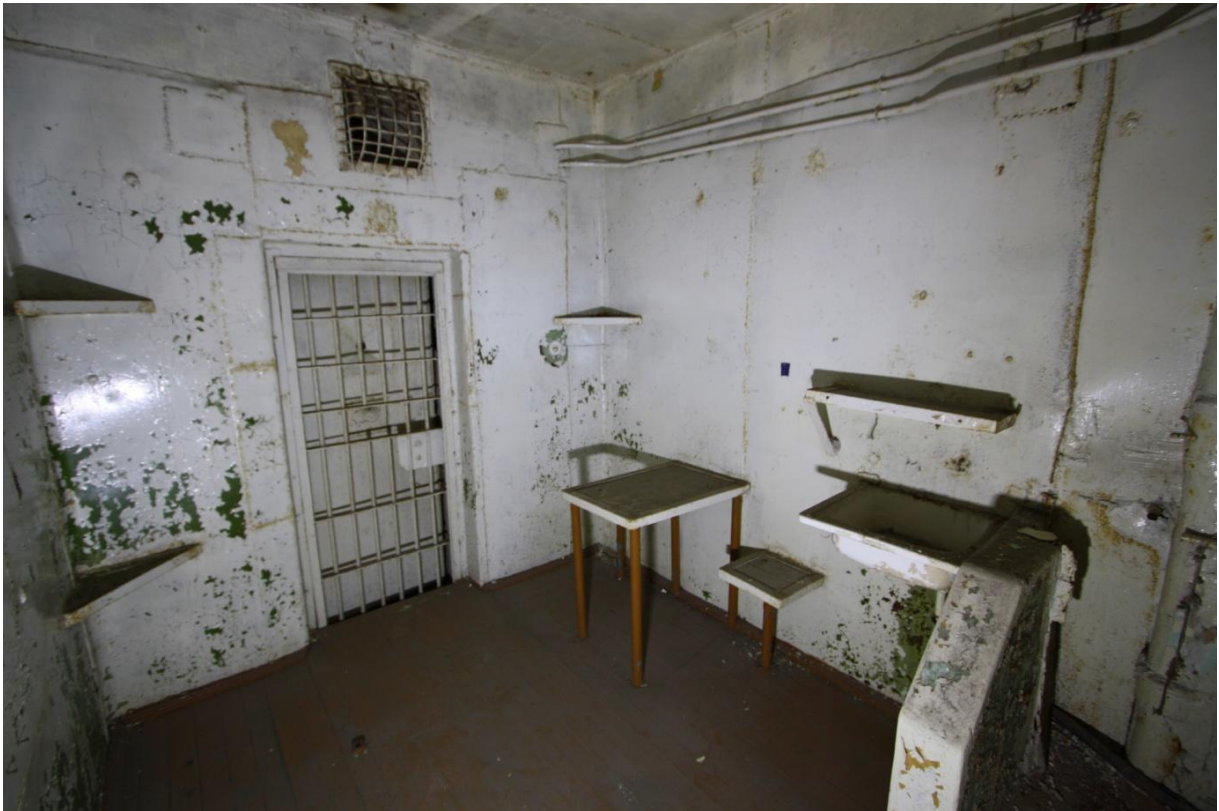
Photo 347. 2 nd floor cell
