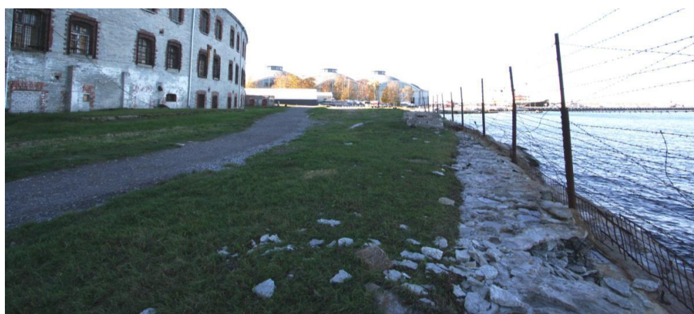
III. 52. View from the east
