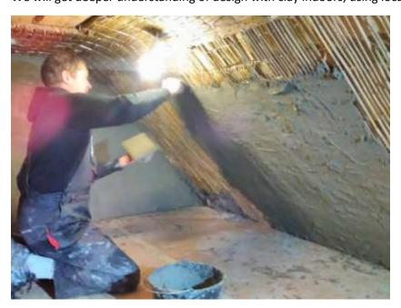
\*Second floor of wooden sauna house, where we work with finishing coats of clay plasters.
