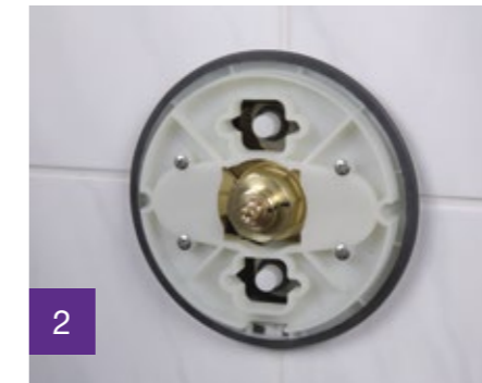
2 Install the mounting plate
