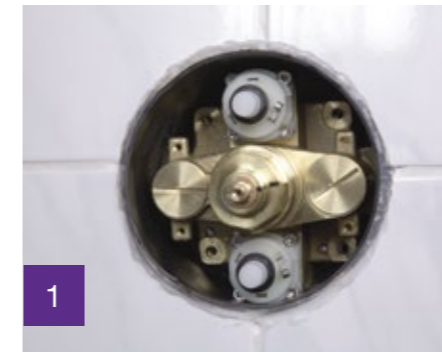
1 Install the functional unit in the KLUDI FLEXX.BOX
