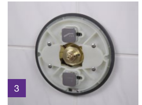
3 Install pushbuttons
