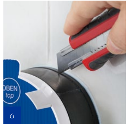
Trim to size – the inside of the box remains protected from dirt during the entire construction phase
