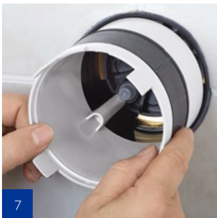
Remove assembly pipe
