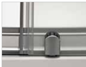
Roller system in the lower part of the enclosure
