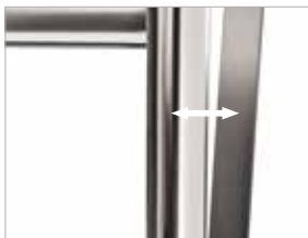
Leveling of wall curves
