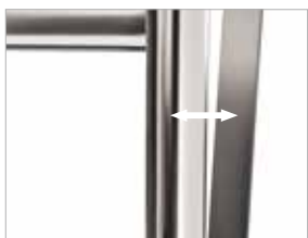
Leveling of wall curves
