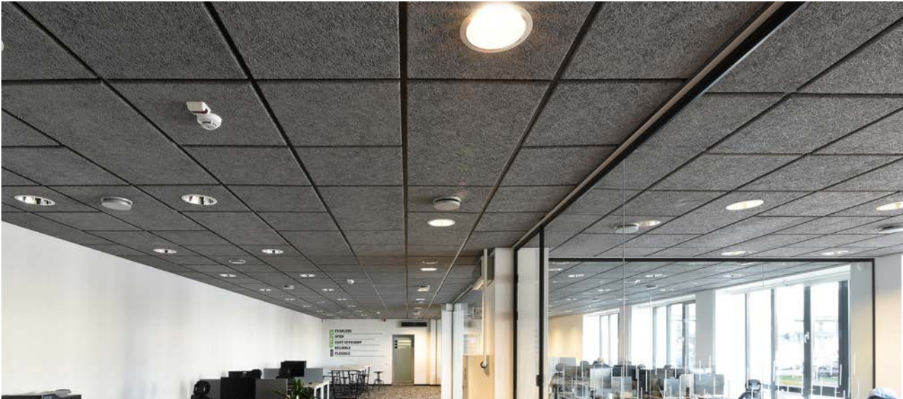
T-type profile frame, P0G edge profile, 25 mm CEWOOD Acoustic panel.
