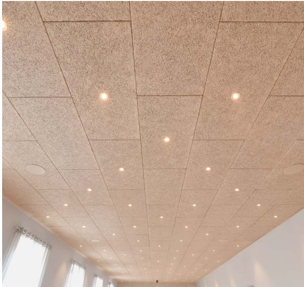
Recessed lights installed into the ceiling
