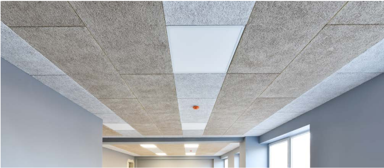
T-type profile frame, P0G edge profile, 25 mm CEWOOD Acoustic panel.
