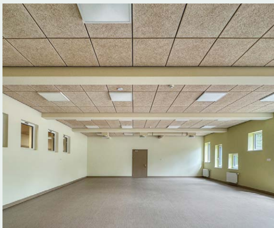
Ceiling finish using CEWOOD panels with a 10 mm gap between each panel.
