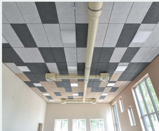
Ceiling finish using CEWOOD panels with a 10 mm gap between each panel.
