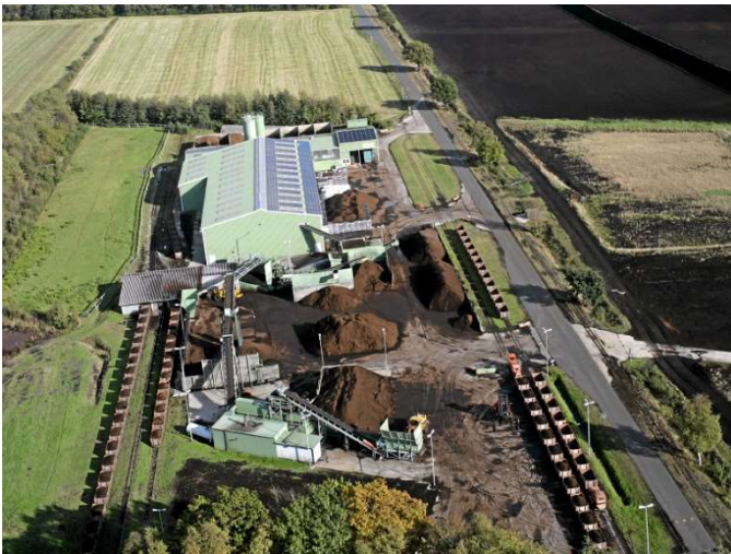
Aerial view of the peat processing plant
