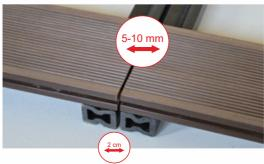
5 At the place where two decking boards collide they each have to end on separate support beam. Available space between support beams. Needed space between support beams at that place is <u>2 cm!</u> The gap between decking boards has to be <u>5-10 mm!</u>
