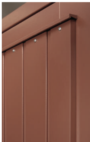
The top of the profile blanking is covered with a timber
