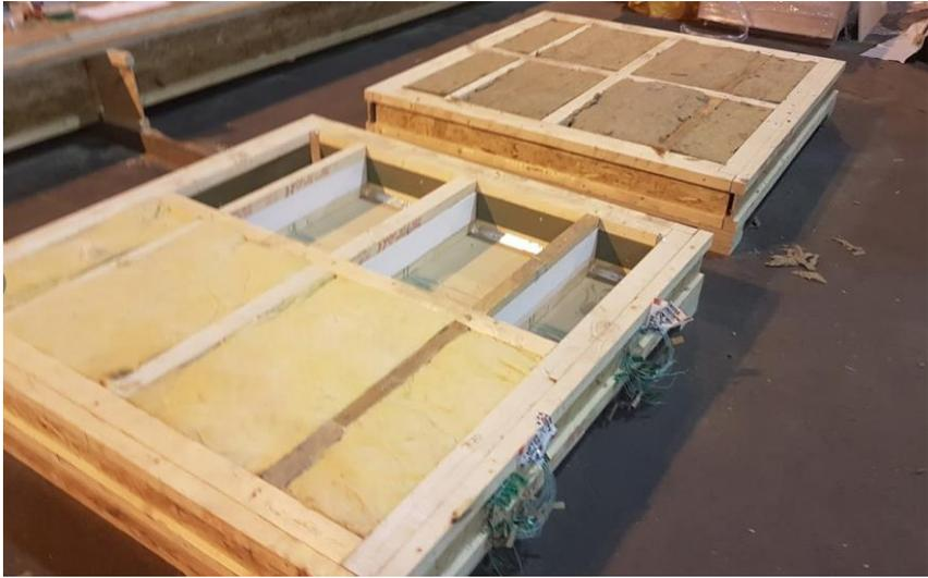
Figure 4.1-7 Construction of the specimen – installing the insulation
