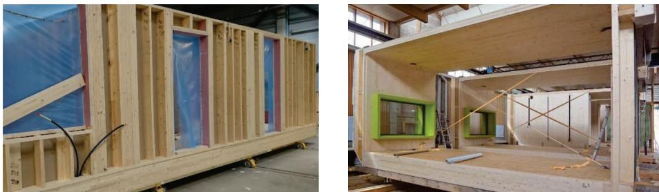
Figure 6. Left: timber frame module; right: cross-laminated timber module (Huß et al., 2018)
