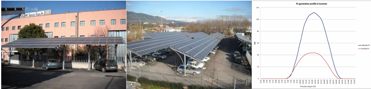
Figure 36. PV plants at the Terni trial site (left) and their production pattern (right)
