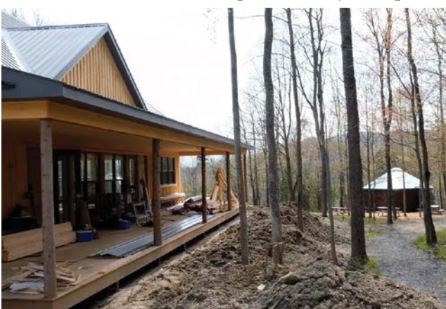
Renovation at Quebec Lodge
