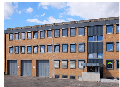
The industrial building at Maschmühlenweg 36 in Göttingen. Microsynth SeqLab is housed on the 2nd floor, where it occupies state-of-the-art lab and office facilities.
