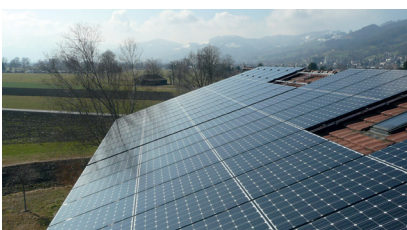
130 m 2 of solar panels capture the frequent sunlight of the St. Galler Rhine valley. This area is known for its above average number of sunny days within Switzerland.
