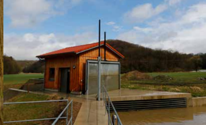
COARSE SCREEN AND VALVE IN INLET
