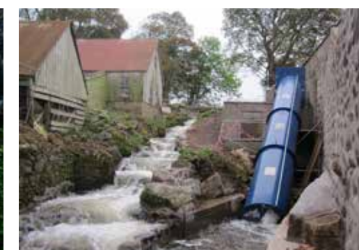
Totally enclosed compact unit (type CR), Haddo, Scotland
