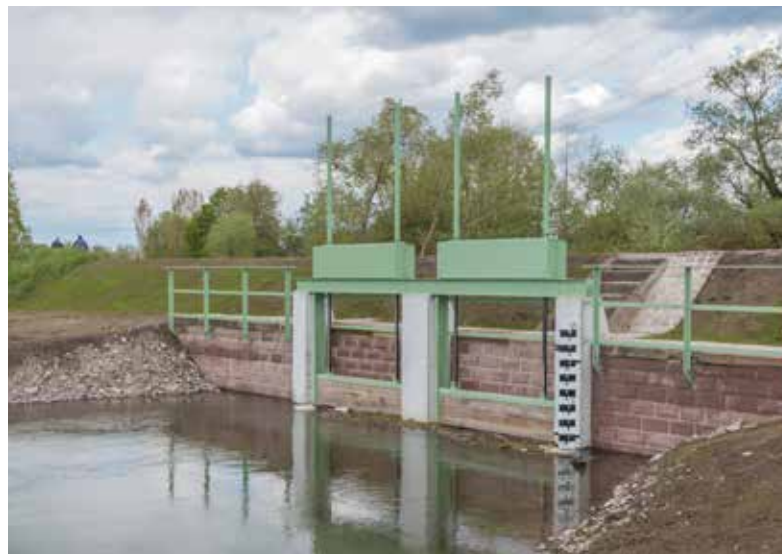
Sluice boards with wooden paneling
