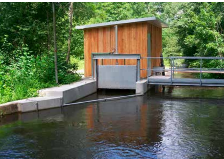
Shut-off valve in front of a hydropower screw
