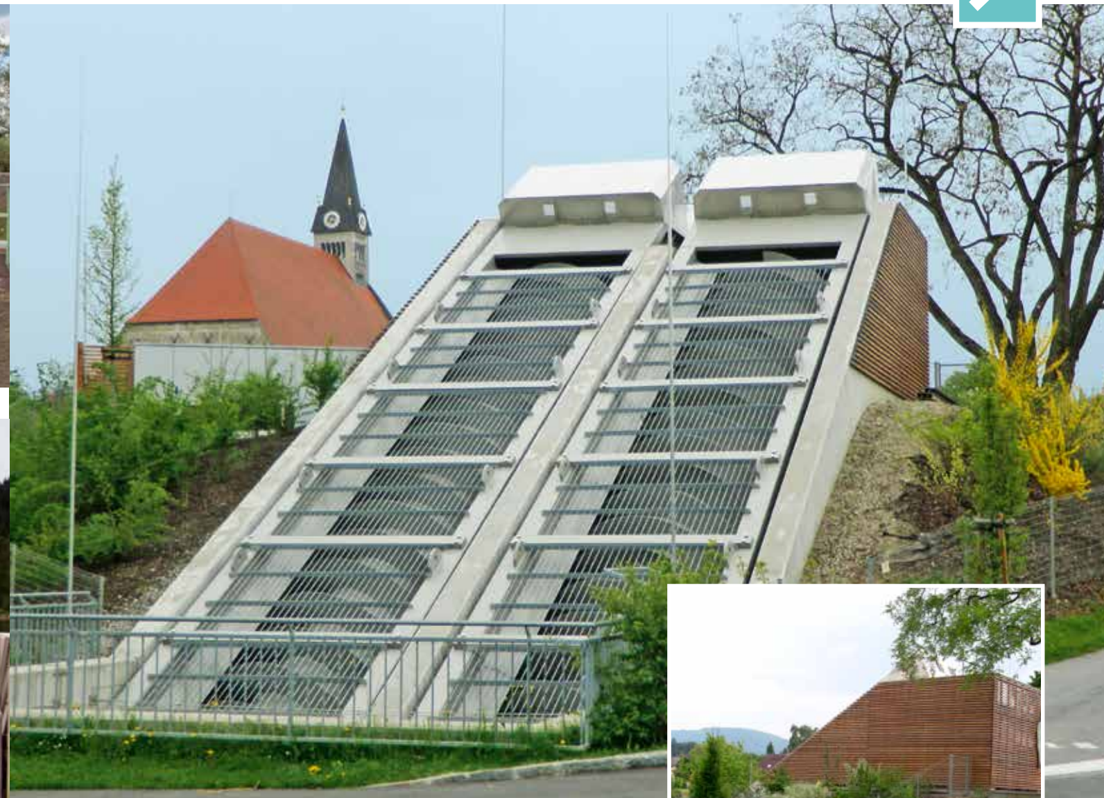
Archimedean screw pump for flood protection in Oberndorf, Austria
