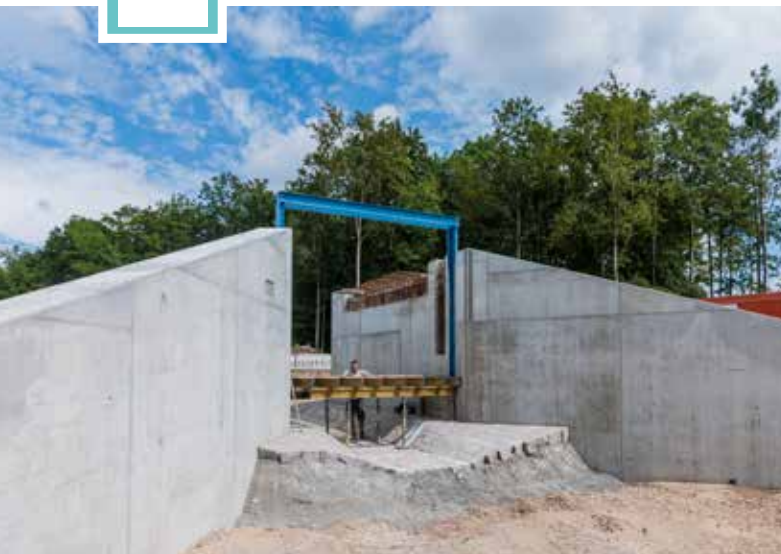
Installation of the guiding frame of a retention gate
