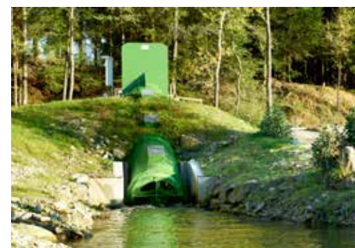
Totally enclosed compact unit (type CR), Bischofsmaier
