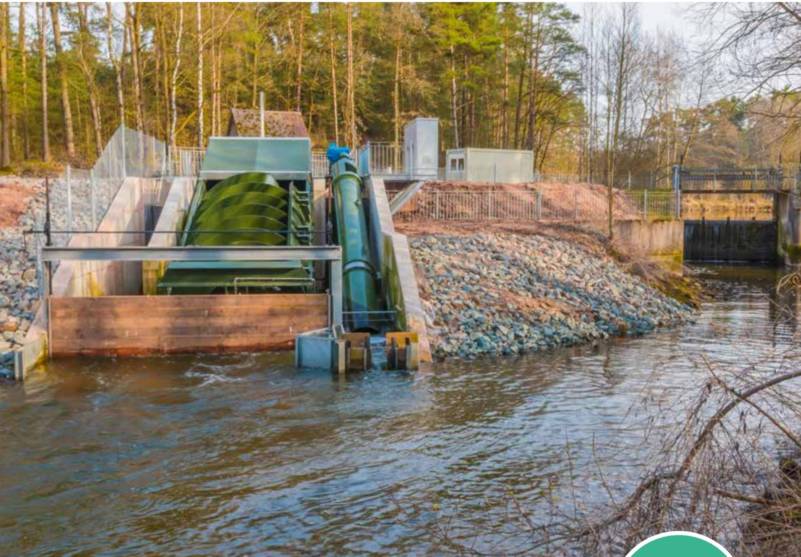
Hydropower screw with fish migration screw at Heckerwehr
