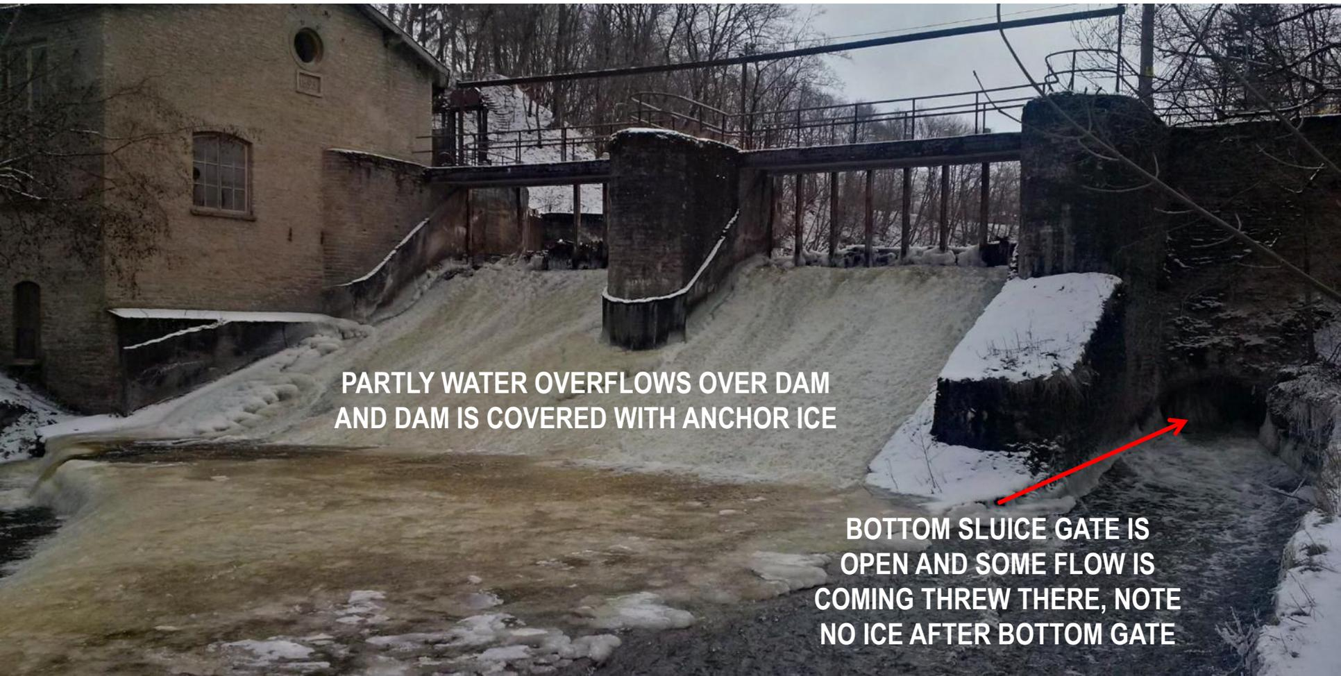
**PARTLY WATER OVERFLOWS OVER DAM
