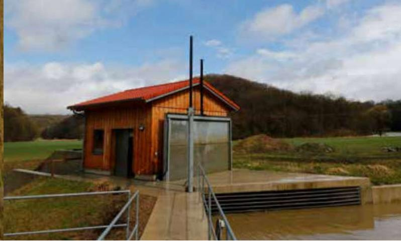
COARSE SCREEN AND VALVE IN INLET
