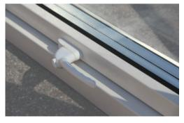
A multi-layered window, the bottom sash is protected with an aluminium glazing bead. To reduce heat loss at the edge of the glass, we recommend using an insulated glazing that has SWS (plastic) spacers rather than the traditional metal.
