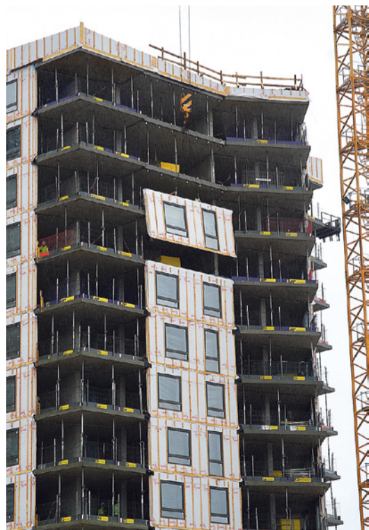
Välisseinaelementide paigaldamine. Foto: AS Timbeco Woodhouse
