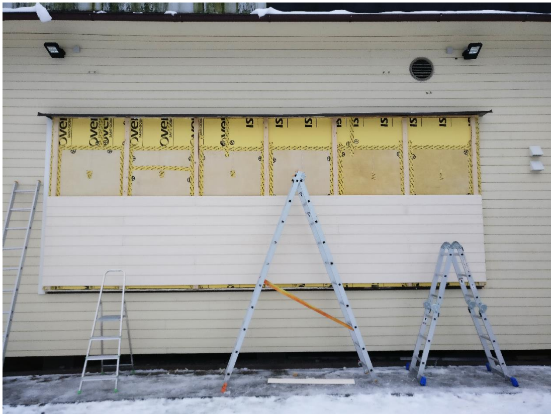
Figure 17. Placement of wall assemblies from outside (Author's photo)
