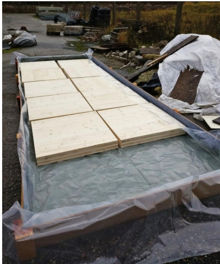
Figure 12. Pool for wetting the CLT panels (Adeniyi, 2019)
