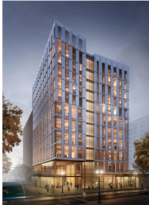
Figure 7. Proposal of 12-storey building of CLT panels, Portland, USA. ( www.dezeen.com , 2017)
