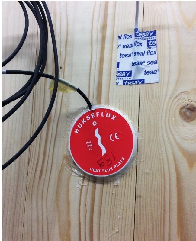
Figure 19. Placement of the heat flux and surface temperature sensors on the inner surface of the test wall (Author's photo)
