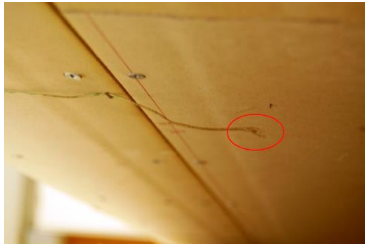
Figure 10 - Thermocouple located on fire exposed side [7]
