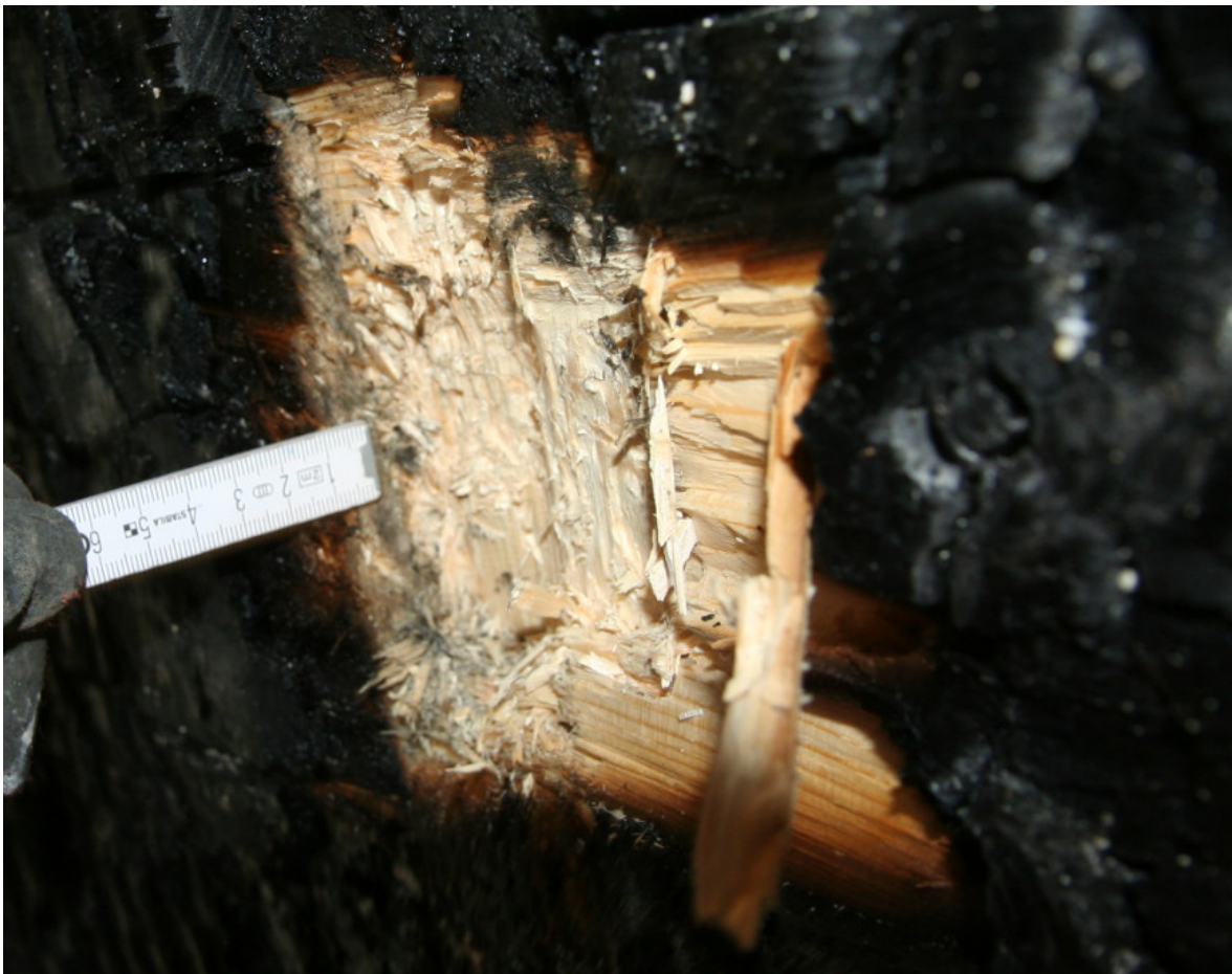
Figure 4.3. Measurements after test showed that approximately 20 mm of the second layer was charred
