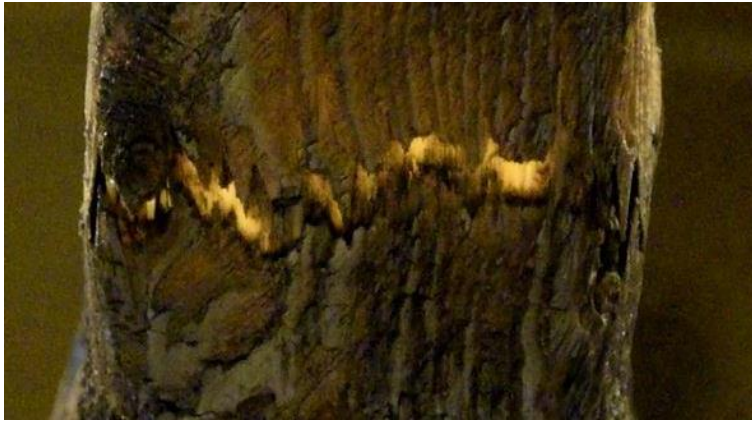
Figure 100. Bottom of the failure zone of Beam 6 after the fire test. Note the fingers of the finger joint.
