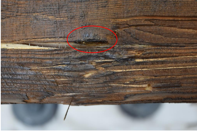
Figure 92. Failure zone of Beam 5 face "B" after the fire test. Note the knot marked with red and clear wood rupture below it.
