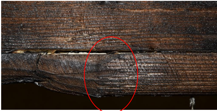
Figure 79. Failure zone of Beam 3 face "B" after the fire test.
