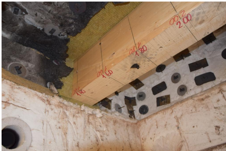
Figure 33. Specimen from inside the furnace before ignition the furnace.
